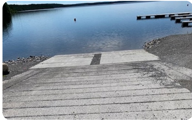
New Launching Ramp
